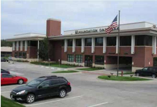
> MOBA Building, 156th & West Maple Road
